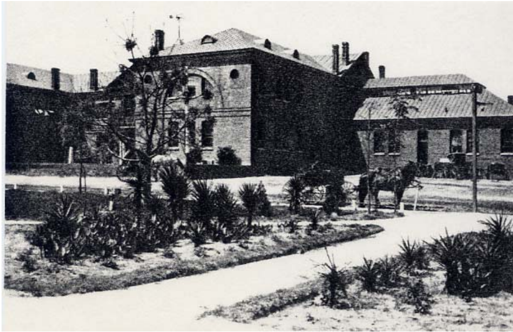
Boys Trades Building ca: 1899 RR Taylor architect lost in a 1918 fire the Willcox Trades Complex replaced this building in 1922 becoming home to Tuskegee Architecture program
